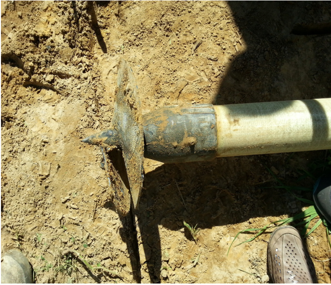
Figure 5. Composite screw pile
