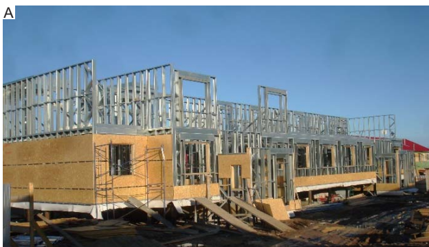
Fig. 1 Installation of the frame for a 16-apartment LSF building in Olenyok settlement (Republic of Sakha (Yakutia)) on screw (A) and pile (B) foundations (from the archive of LLC “Adgezia-MK”)
