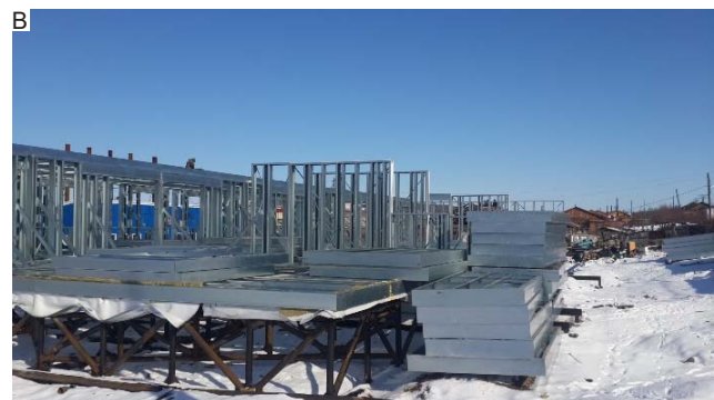
Fig. 1 Installation of the frame for a 16-apartment LSF building in Olenyok settlement (Republic of Sakha (Yakutia)) on screw (A) and pile (B) foundations (from the archive of LLC “Adgezia-MK”)
