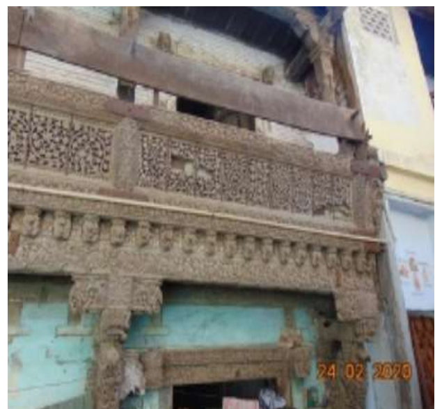
Fig. 7. Façade with wooden carving (Source: Gangwar and Kaur, 2020)
