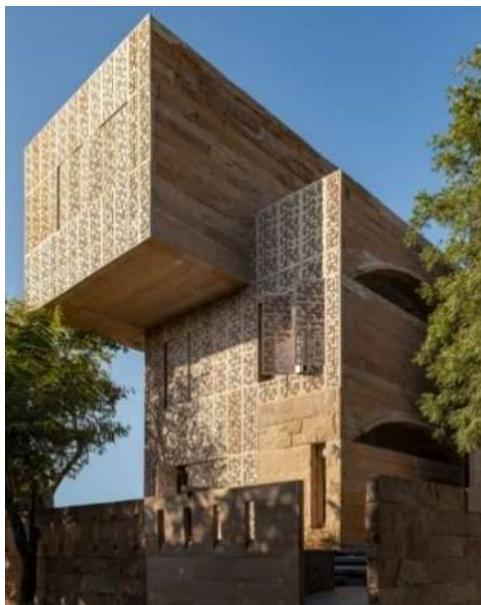
Fig. 17. View of stone house
