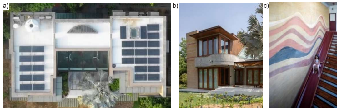
Fig. 25. Roof top solar panels (a), Large overhangs (b) and Rammed earth wall (c)
