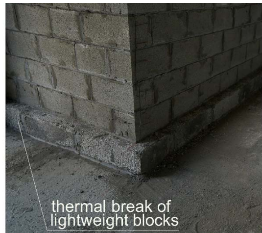
Fig. 3. Thermal break in masonry with the use of lightweight blocks
