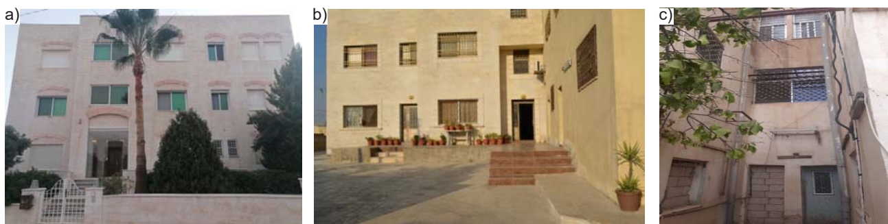
Fig. 1. Main facades of the buildings of different forms: (a) rectangular, (b) L-shaped, and (c) U-shaped
