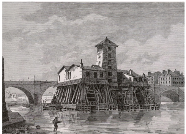
Fig. 6. Pompe Notre-Dame (Notre-Dame Pump) originally built in 1670 and reconstructed in 1708. This pump raised waters from the Seine into many public fountains and monuments, and it is said that it would allow the fountains to shoot water from 12 up to 50 feet in the air. Here shown in 1861, the pump looks rather destitute and neglected next to the Pont-Notre Dame. The Pont underwent much renovation during the 19 th century, while the pump itself remained virtually untouched (source: https://fr.wikipedia.org/wiki/Fichier:Pompe_Notre-Dame,_vue_prise_de_la_vo%C3%BBte_du_quai_de_G%C3%A0vres_en_1861.jpg )
