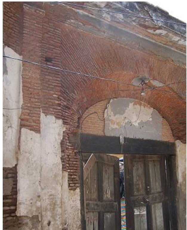
Figure 9. Thick masonry of lakhauri bricks in traditional houses (Source: the author of the paper)
