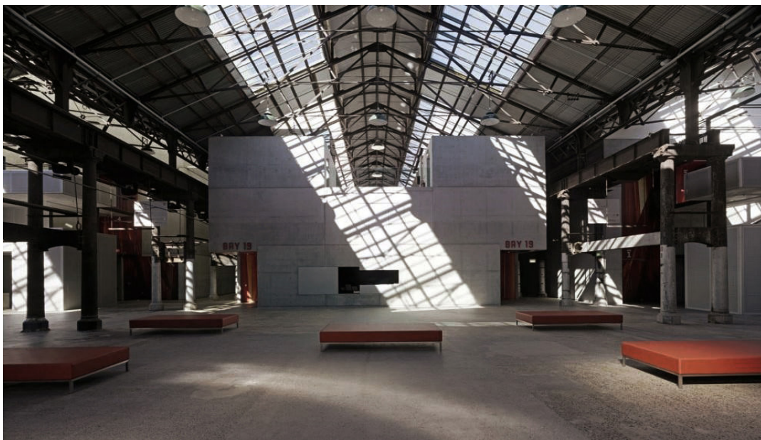
Figures 5–8: Transformation of the abandoned Eveleigh Rail Yards, built in Sydney, Australia, in the 1880s, into Carriageworks, a modern center for performing arts (theater, experimental dance, acrobatic shows)
