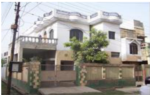
Figure 24. Front view of the contemporary LDA House (Source: the author of the paper)
