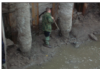
Figure 4. Pile construction using the Fundex technology (a) and a necking defect along the length of the pile shaft (b).
