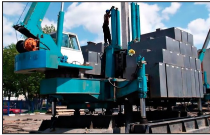
Figure 3. Pile construction by jacking.
