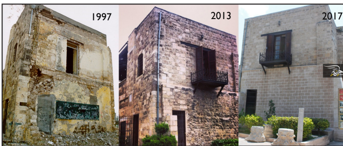
Figure 9. Southern building of the Pasha’s Palace complex before and after restoration (Mitri Abu Aita, 2004).
