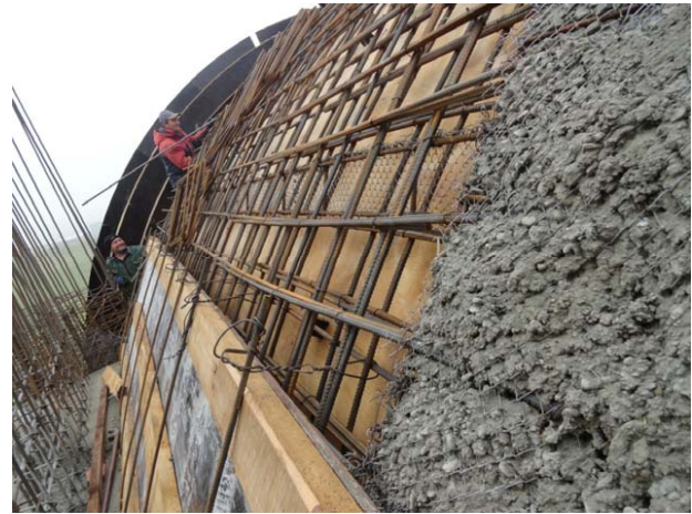
Fig. 8. Assembly of the flexible external mold
