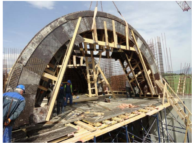
Fig. 4. Transportation of the arched beam molds
