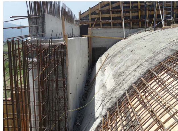
Fig. 9. Concreting of the shell roof
