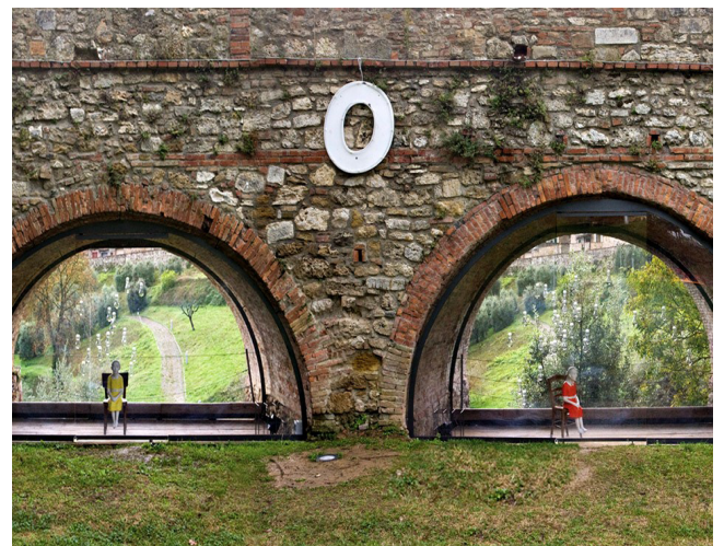
Figure 47. A bridge is used as an art gallery (Colle Val d'Elsa)
