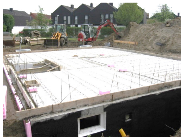
Figure 7. Precast reinforced-concrete ceiling with in-situ concrete added. Photo by D. Mähner
