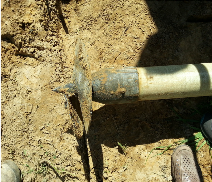
Figure 5. Composite screw pile
