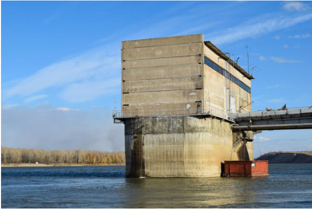
Figure 2. Water intake facility on the Tom River
