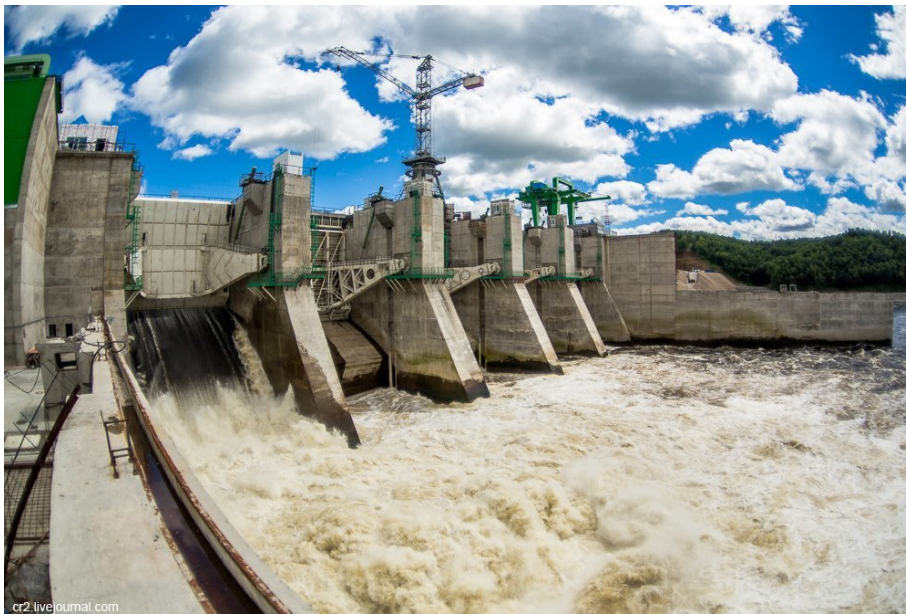
Figure 4. Water intake with diversion weirs at the Bureya hydroelectric power plant ( https://fishki.net/2603030-sejchas-stroitsja-v-rossii-post-nomer-19-nizhne-burejskaja-gjes.html )
