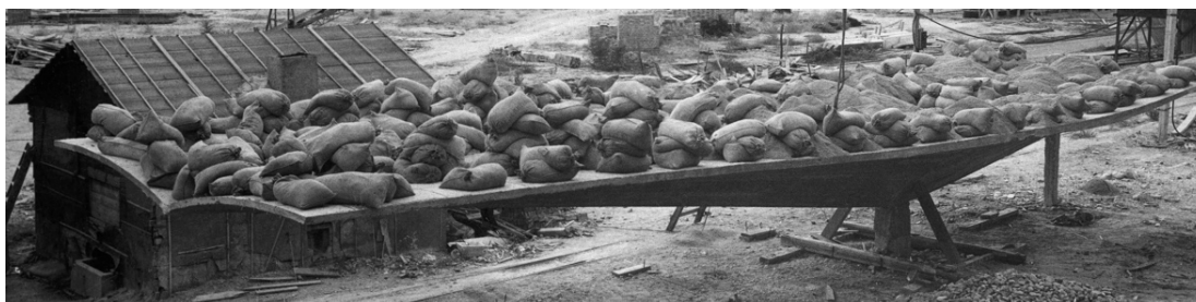
Figure 9. Load test of the cantilever module (archive: Eduardo Torroja)
