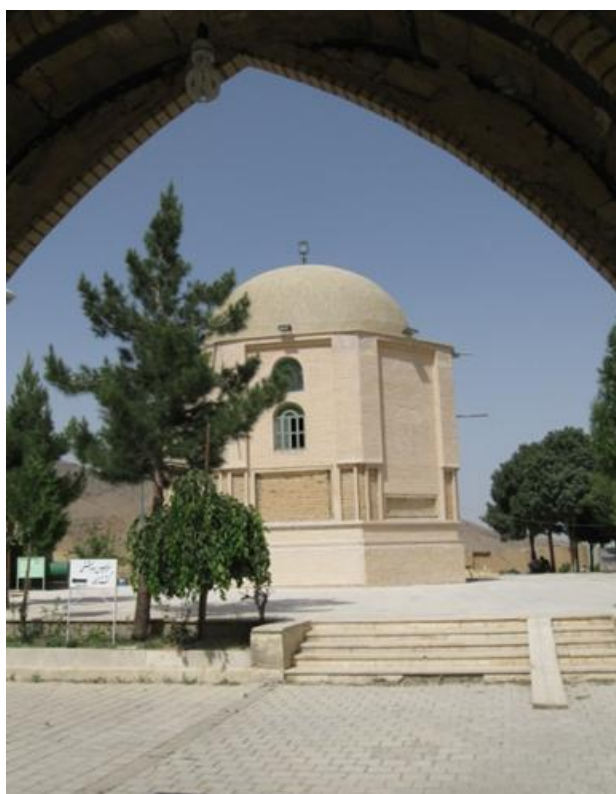
Fig. 2. A landscape view of the Imamzadeh Abdullah building (Photo by A. Moghaddasi)
