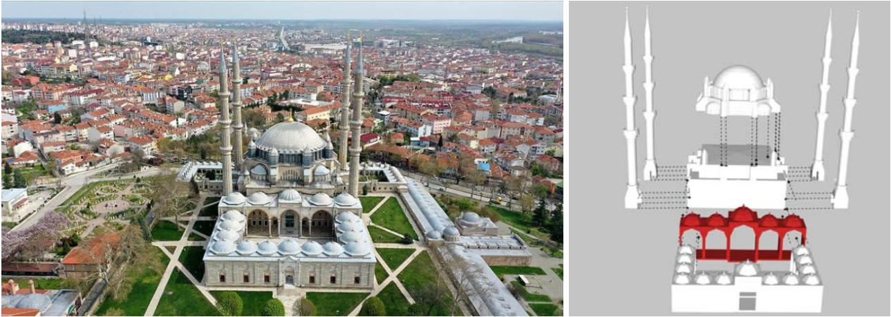
Fig. 3. Front view of the Selimiye Mosque in Edirne and model of the mosque parts and the narthex (TRT News, 2025; revised and remodeled by the corresponding author)
