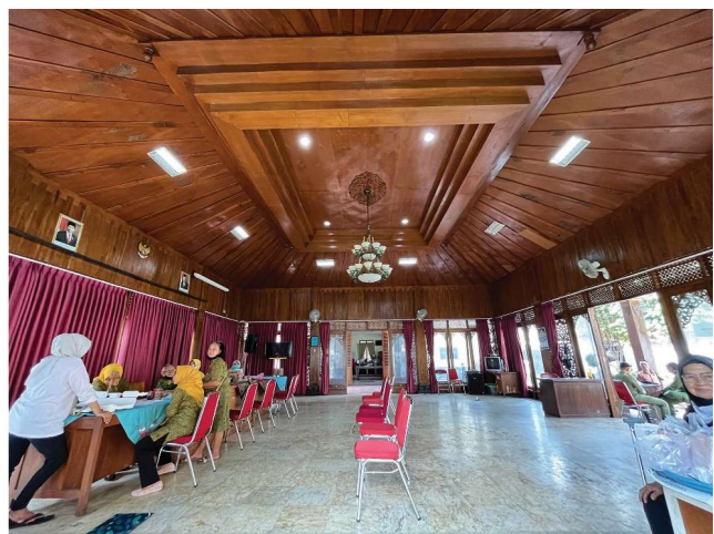
Fig. 4. The interior of public halls showing the use of 'wooden' materials. Some use saka guru and tumpang sari (left), while others only use tumpang sari without saka guru (right) revealing that those features are just ornaments. The materials used are usually concrete, with wooden tiles to make an impression of wooden posts/beams. Photos by author
