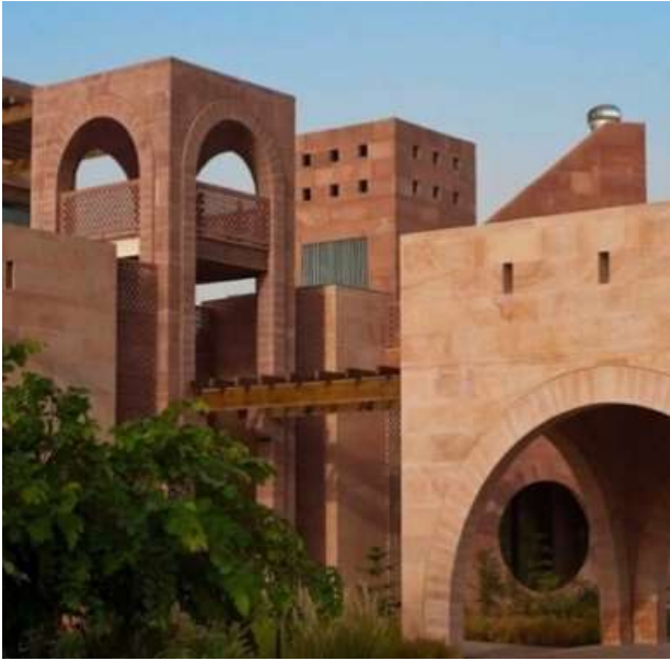
Fig. 12. Entrance of Shunyam residence (Source: archiol.com)
