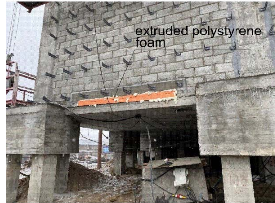
Fig. 2. Thermal break in masonry with the use of a perforated beam
