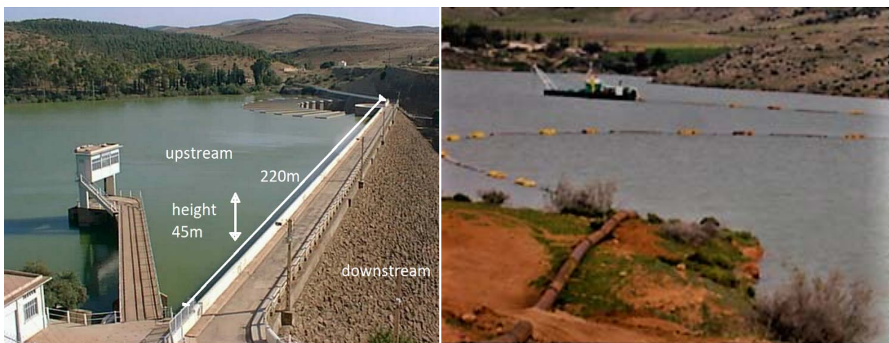
Fig. 1. View of the reservoir of the Bakhadda dam and the Djebel Debbagh stationary dredger
