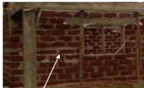
Fig. 1. Illustrations of the components of the adobe brick masonry units for the Brick Building: (a) individual sun-baked brick unit; (b) typical constructed walls joined with cement-sand mortar (images adopted from: Abanda et al., 2015).
