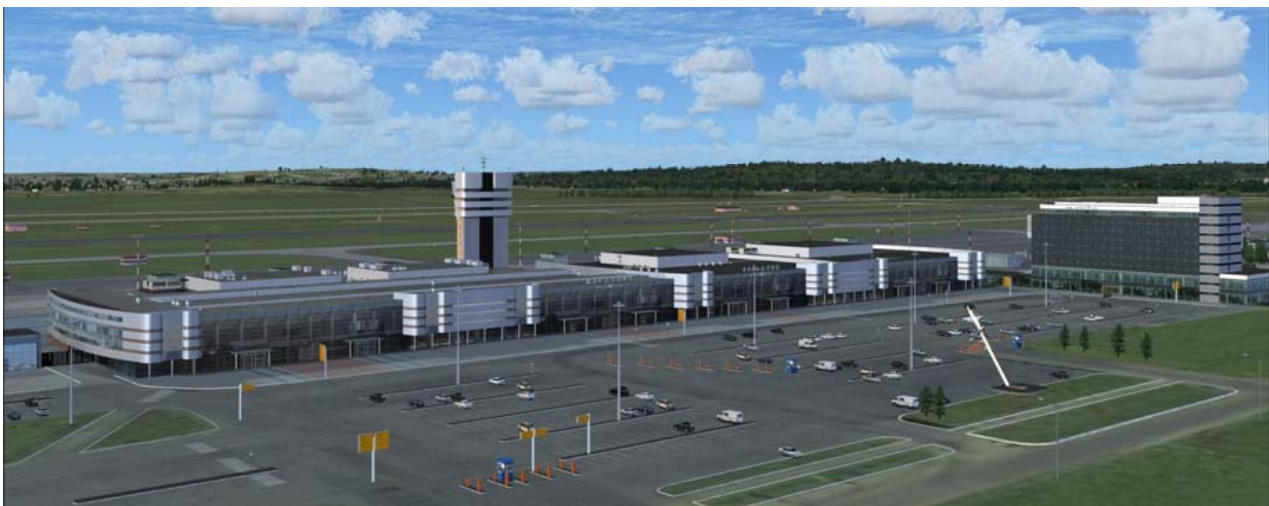
Fig. 1. Long airport complex building
