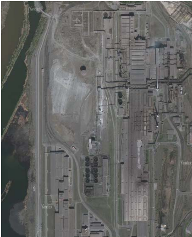
Fig. 3. Chimney as part of the coke oven complex
