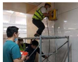
Detection with a ground penetrating radar
