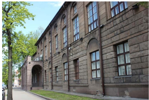
Fig. 3. Fragment of the north-eastern facade of the State Bank, Yaroslavl
