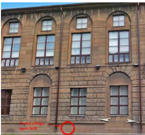
Fig. 5. Location of material sampling from the building of the Yaroslavl Central Bank
