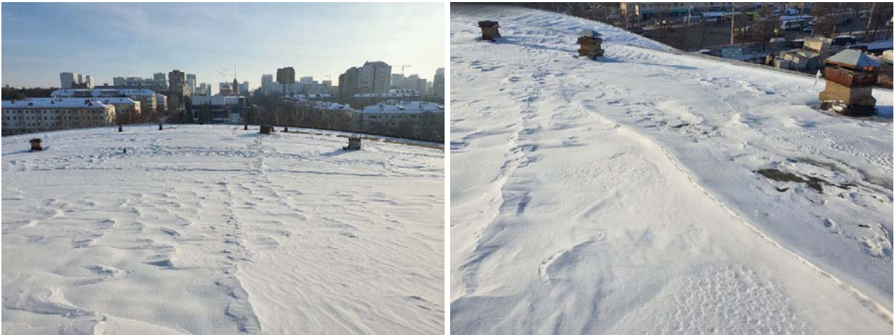
Fig. 4. Photo recording of snow transfer on a full-scale facility
