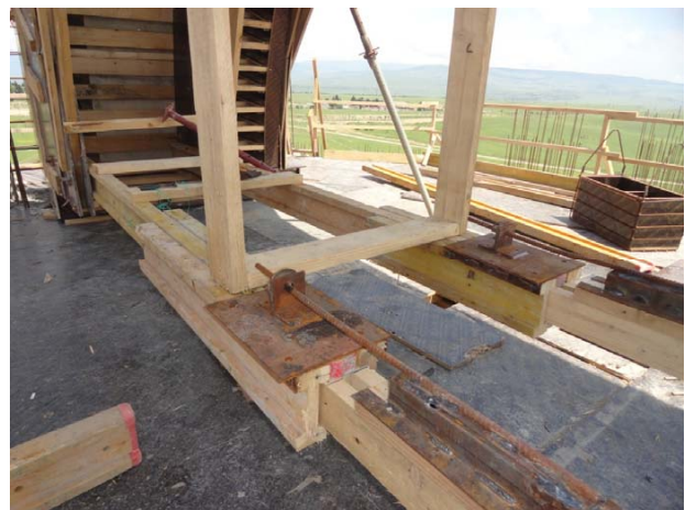
Fig. 5. Movable lower assembly of the arched beam mold
