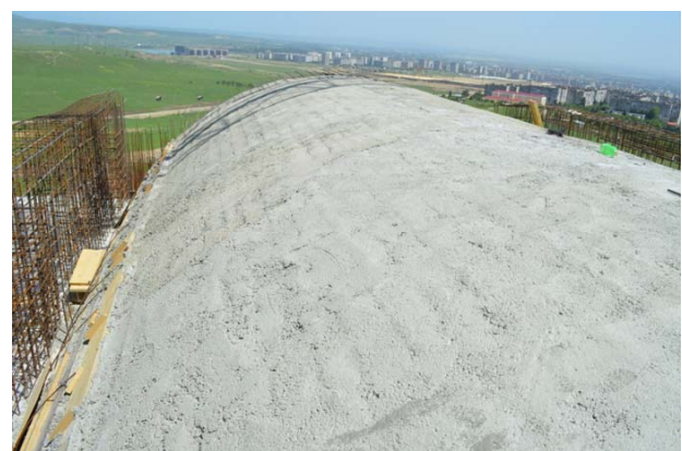
Fig. 10. Finished shell roof
