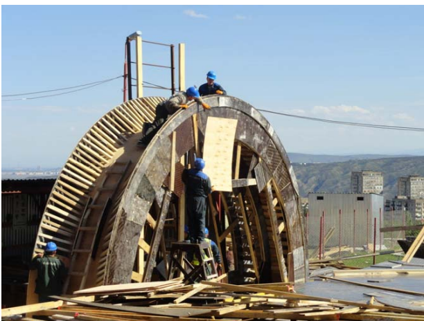
Fig. 3. Assembly of the arched beam molds
