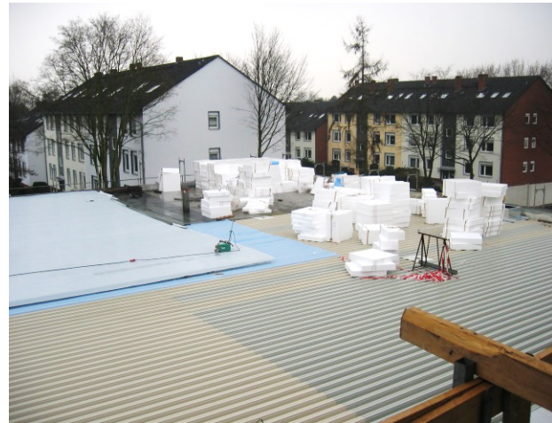
Figure 9. Non-ventilated flat roof. Photo by D. Mähner
