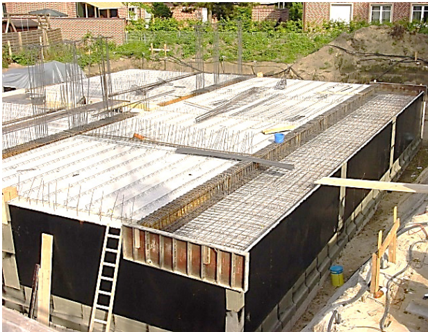
Figure 8. Precast reinforced-concrete ceiling with in-situ concrete added. Photo by D. Mähner
