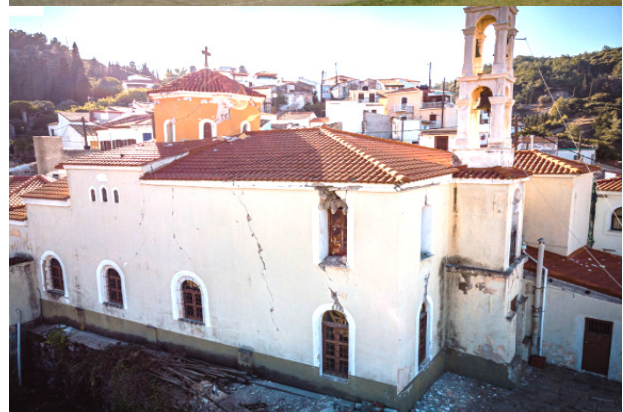
Figure 17. Typical damage to the peripheral masonry walls of "Basilica" churches from earthquake activity in Greece. At the top, a "Basilica" church at the village of Nisi from the Patras-Pyrgos earthquake of 8th June, 2008. At the bottom, a "Basilica" church at Karlovasi damaged from the Samos earthquake of 2020 (Manos and Kozikopoulos, 2015; Manos, Soulis, Karamitsios, 2012; Manos and Karamitsios, 2013; Manos, 2016; Manos, Kotoulas and Kozikopoulos, 2019; Manos and Kotoulas, 2019)
