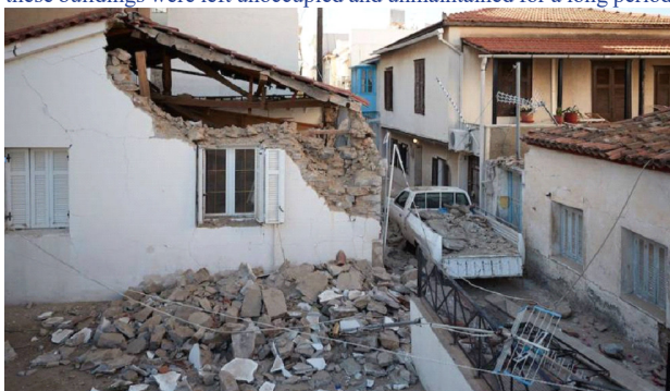
Figure 24. The partial collapse of old unreinforced masonry structures at Vathi that caused the death of two young teenagers
