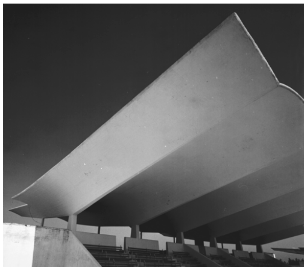
Figure 8. Cantilevered shells (archive: Eduardo Torroja)
