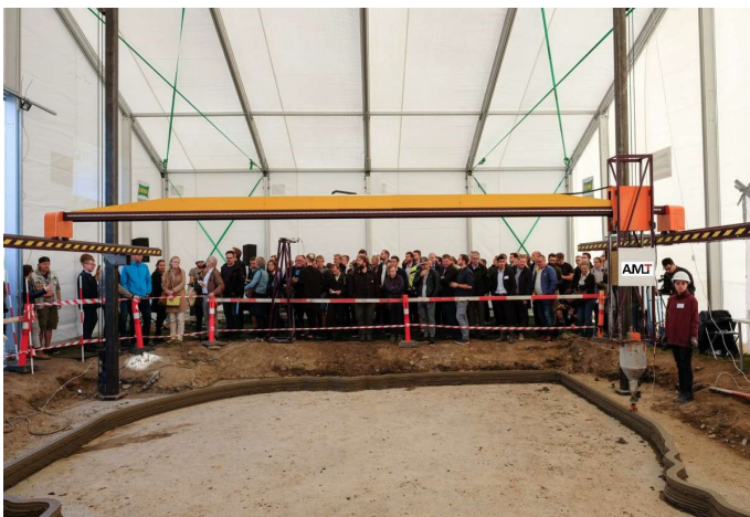
Figure 3. AMT S-6044 LONG2 construction 3D printer.
