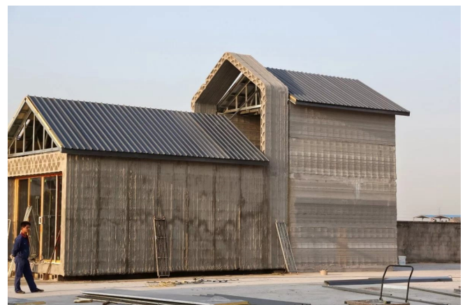
Figure 2. Assembled building at a construction site.
