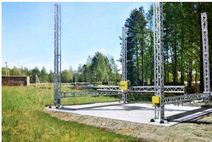
Figure 4. AMT S-300 construction 3D printer.
