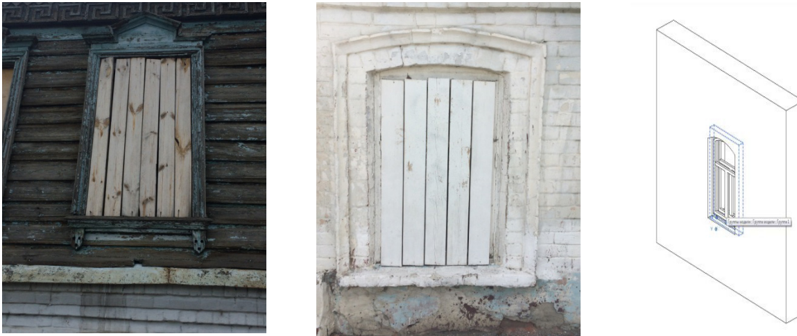
Figure 6. Examples of unique elements of a building as a part of an actual cultural heritage site and BIM model. Source: photo by the authors, BIM model.
