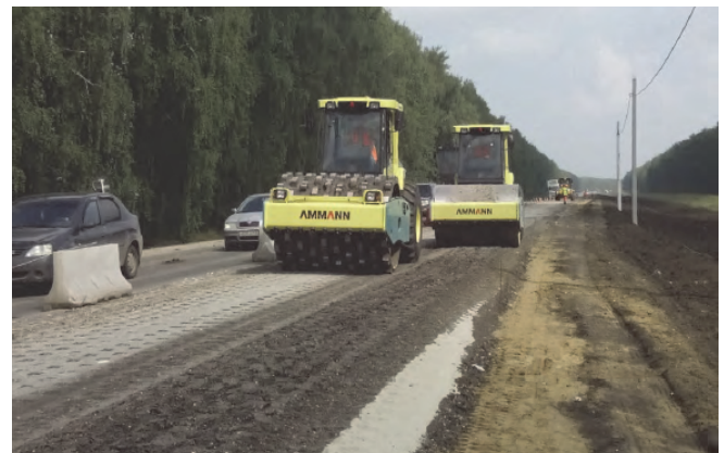
Figure 7. Cold recycling with addition of foamed bitumen, cement and granulated slag (Federal Road Agency (Rosavtodor), 2016)
