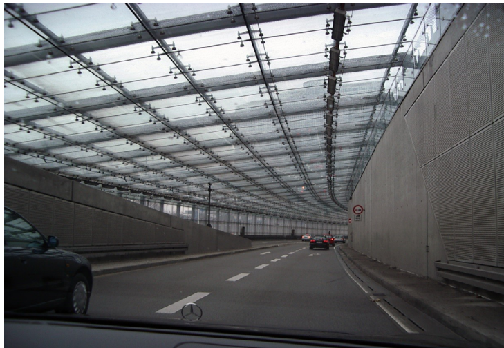
Figure 7. Translucent roofing in the Petuel Tunnel (Munich)
