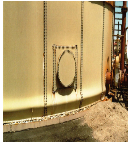
Elephant foot bulge during the May 1983 Coalinga Earthquake
