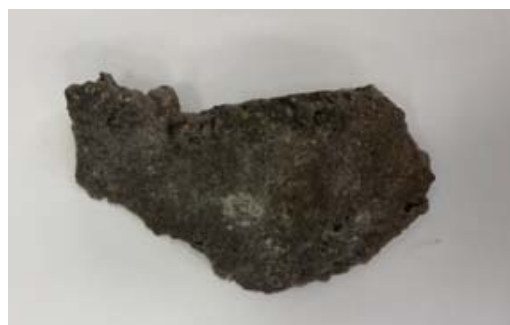
Fig. 8. Sample No. 2 of the plaster of the Main Treasury building in St. Petersburg
