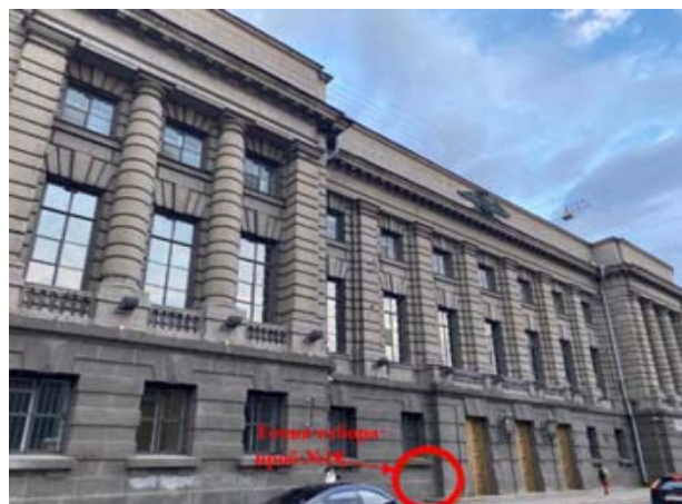
Fig. 7. Location of material sampling from the Main Treasury building in St. Petersburg
