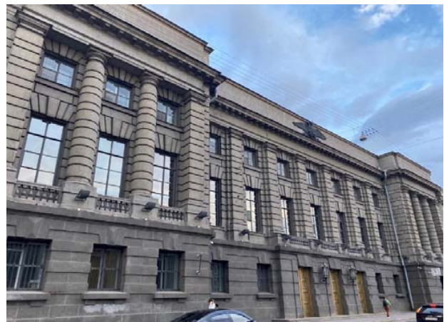
Fig. 4. View of the main facade of the Main Treasury, St. Petersburg
