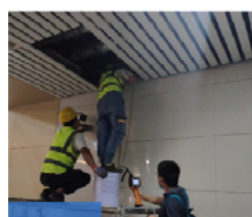
Inspection with an industrial endoscope
