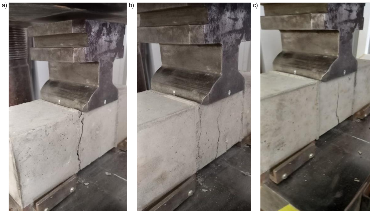
Fig. 4. Cases of specimen fracture when determining the shear strength of concrete: (a) by shear stresses (“pure shear” according to Stolyarov (1941)); (b) by shear and normal stresses (“shear” and “bending”); (c) by normal stresses (“bending”)
