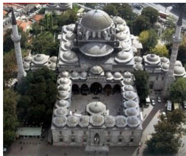
Fig. 5. Roofing of the mosque
