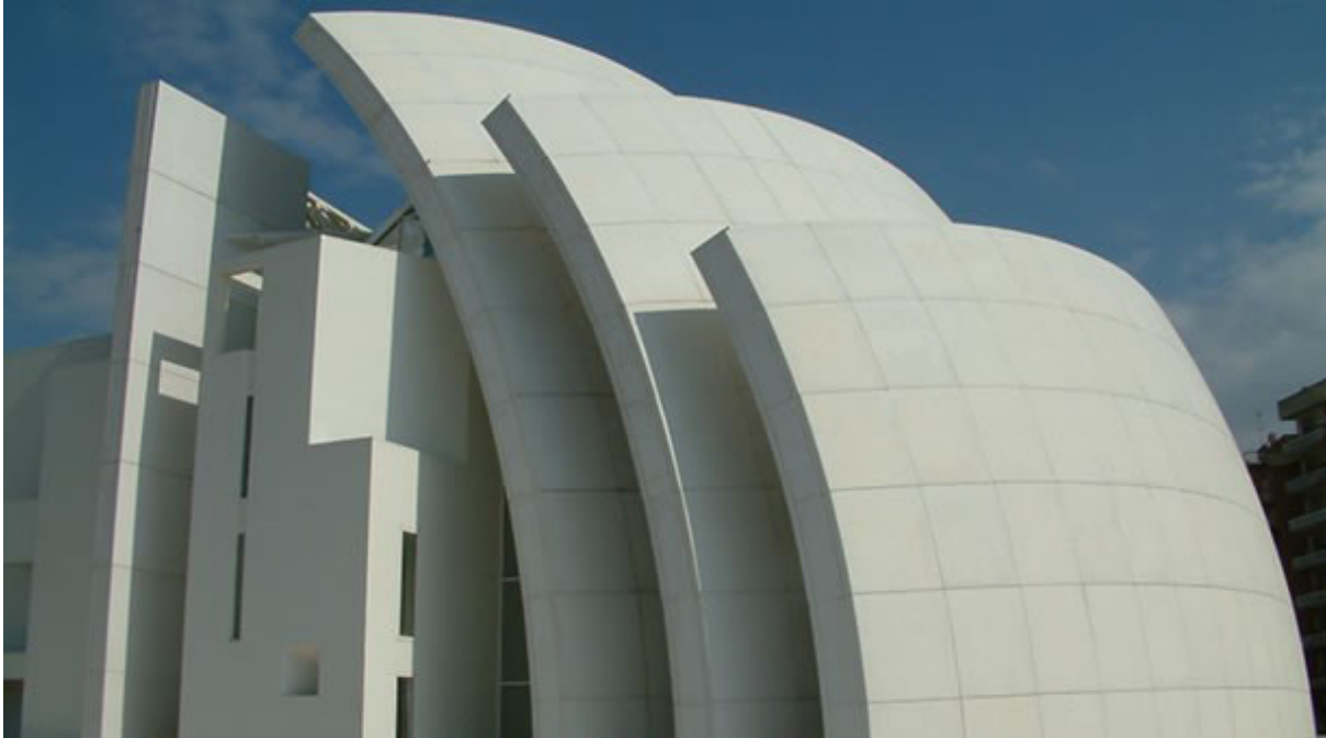
Photo 1. The church made from self-cleaning concrete always keeping its whiteness, "Rich in Mercy", Dives in Misericordia, Rome.
