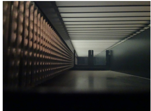
View inside the convector enclosure
