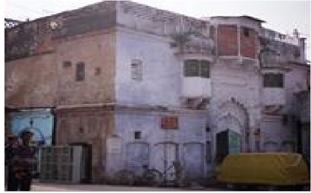
Figure 11. Exterior view of Rizvi House (Source: the author of the paper)
