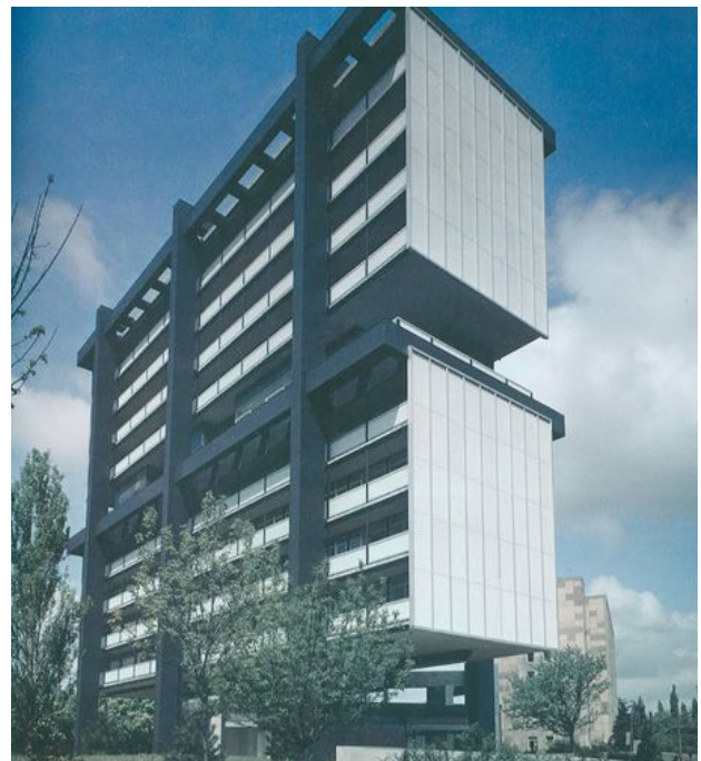
Figure 7. Maison de l'Iran, Paris, France (Hidden Architecture website: http://hiddenarchitecture.net )
