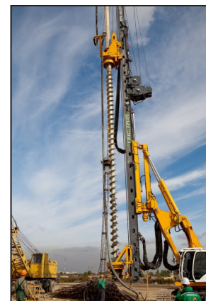
Figure 6. Pile construction using the CFA technology.
