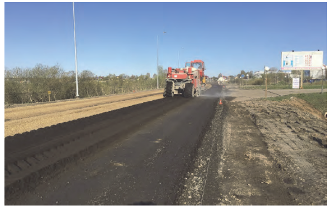
Figure 6. Cold recycling using WR-2500 Wirtgen recycler machines (complex binder: bitumen emulsion, cement) (Federal Road Agency (Rosavtodor), 2016)
