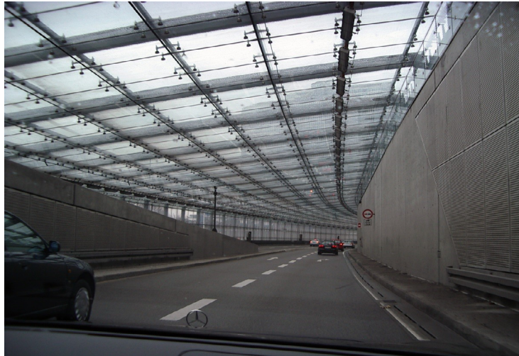
Figure 7. Translucent roofing in the Petuel Tunnel (Munich)
