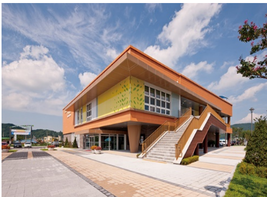
Figure 2. Community centre at Asan City
