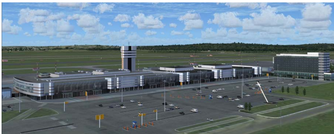
Fig. 1. Long airport complex building
