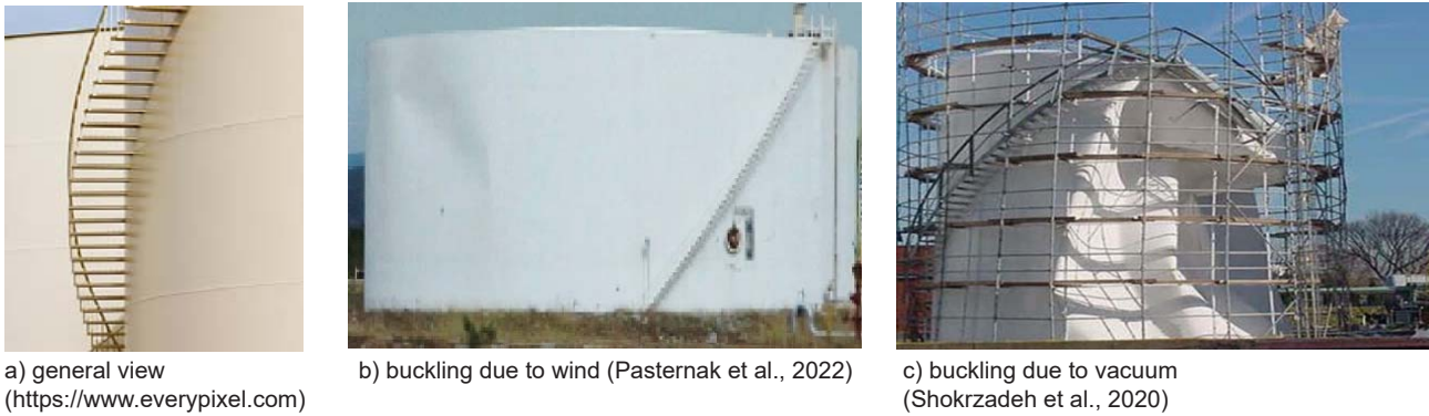
Fig. 3. Tanks with technological stairs
